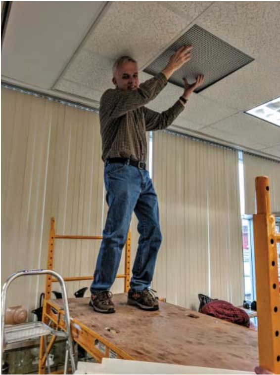
Greg Vass climbed up on the scaffolding to remove the ceiling vent for cleaning.
